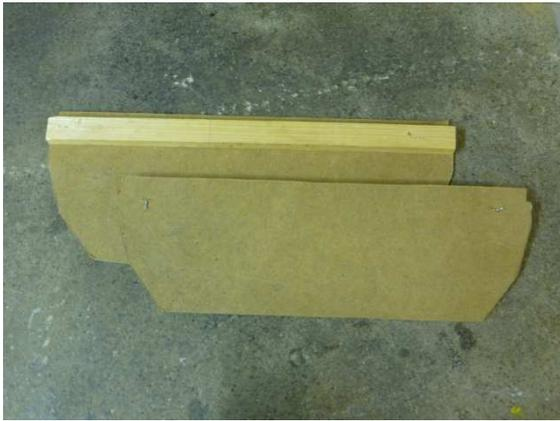
Cut roof battens to correspondingly long pieces. To temporarily connect the wooden battens lengths to the moulds, drill two 2 mm holes close where the batten ends. Pull wires through and twist them together.
