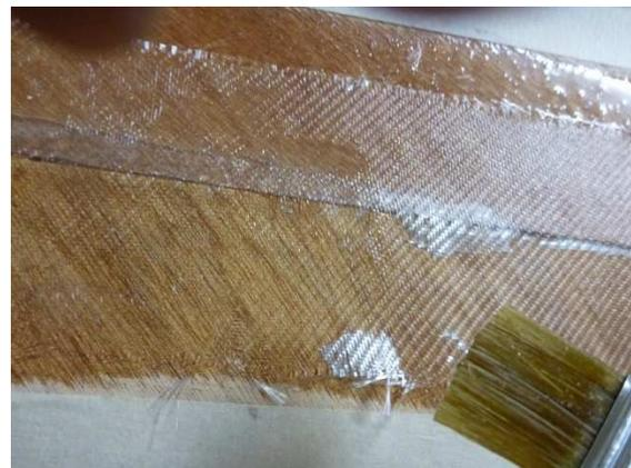
In the picture above this text two sections are visible where the glass fabric remained white. Here, apply a small additional amount of epoxy with the brush until the areas are transparent. In the picture below this text, all places are saturated with epoxy.
