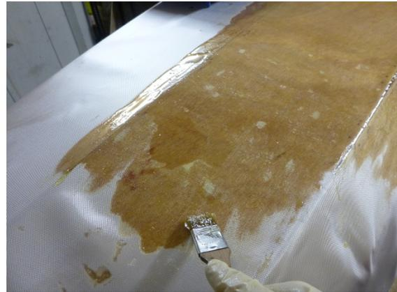
..., do not worry about bubbles, peaks and puddles, just keep working. After a few minutes the tissue and the underlying wood is wet. The epoxy is soaking into the glass and the wood. Now apply some more epoxy and brush or roll the last air bubbles away:
