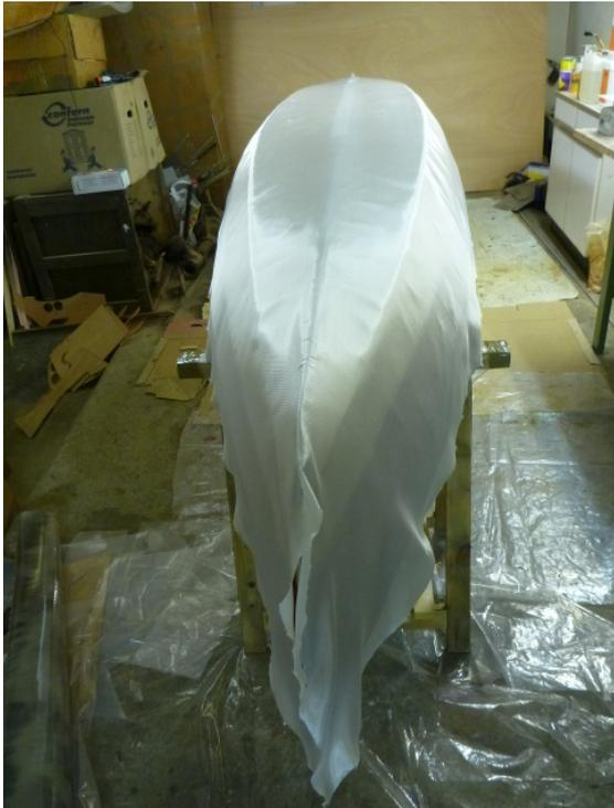
At the coaming, the glass cloth is cut about 10 cm from the edge. The remains of glass fabric are not thrown away! We will need them later for the deck reinforcements!
